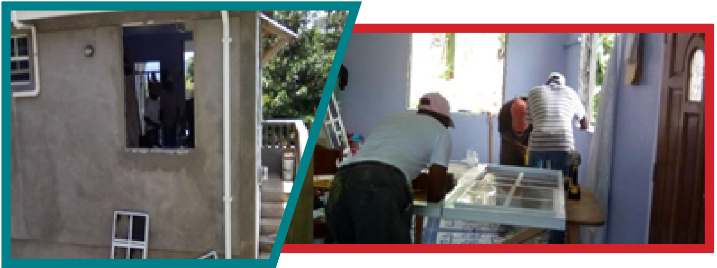
REPLACING DAMAGED WINDOWS AT SALISBURY
